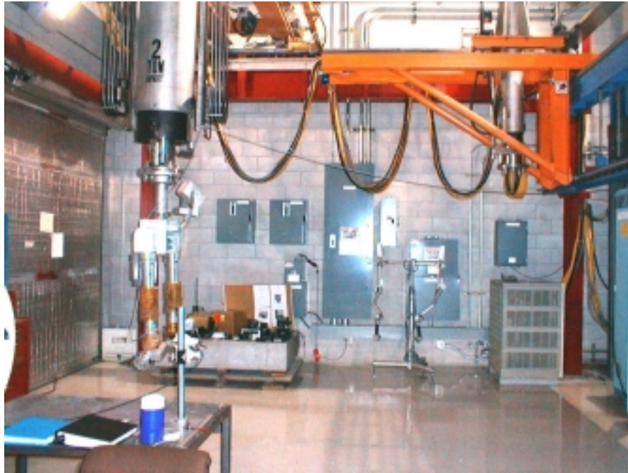
Figure 1. Robotic Hot Cell Unit in UNLV's Robotics Lab. This large work cell (approx. 20 x 20 ft floor space) features two large gantry robots with 1- and 2-ton lifting capacities. The large robot is equipped with a tool changer for various attachments, including a remotely controlled master-slave dual arm end effector.
